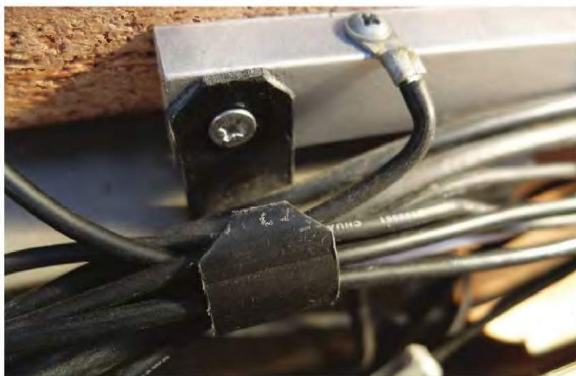
PHOTO 3: A finished J-clip, cable bundle and earthing point.
